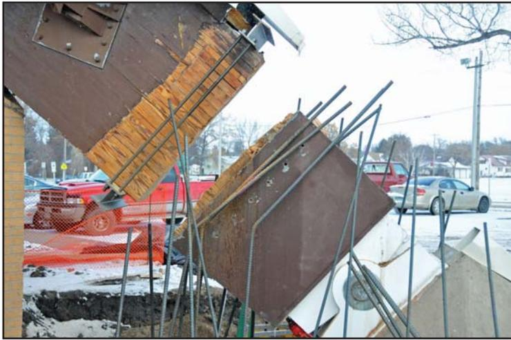
With the shoring towers in place, the bases of the arch could be completely removed and repairs made.
